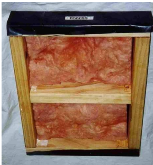
Figure 4: Inoculated unit prior to fixing building paper and fibre cement cover
