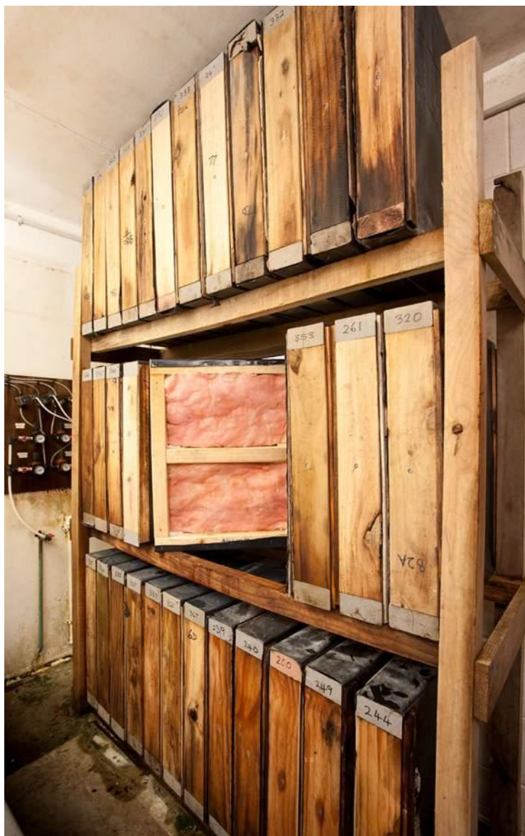
Figure 5: Frame units in controlled environment room (cover removed from one)
