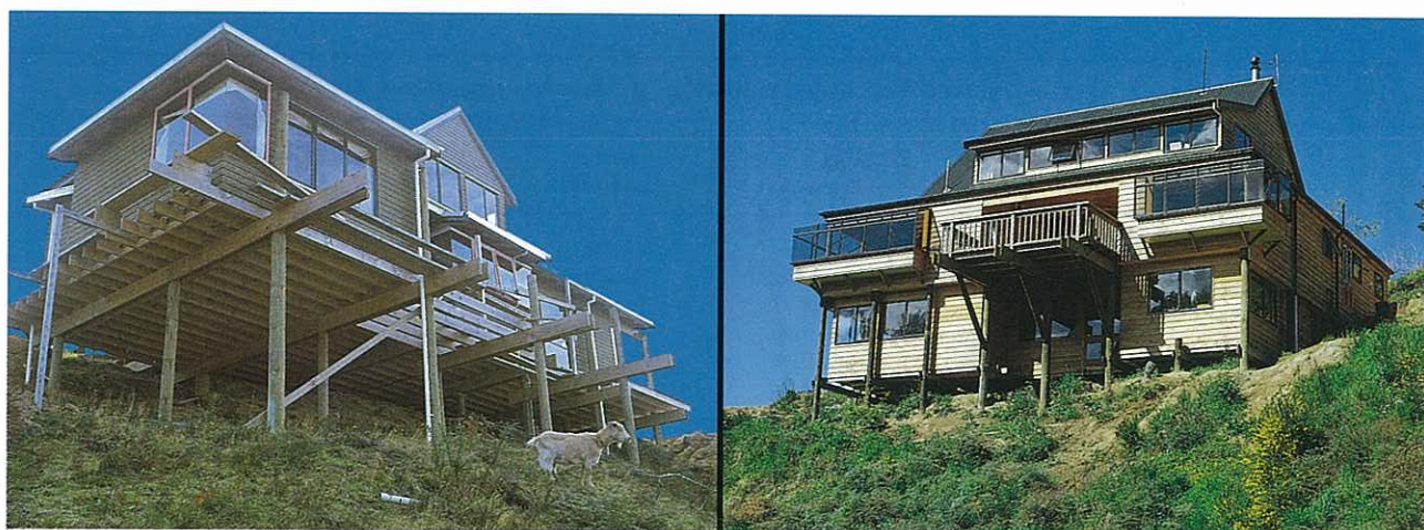
Houses clad with preservative-treated radiata pine (left), and naturally durable macrocarpa (right).
