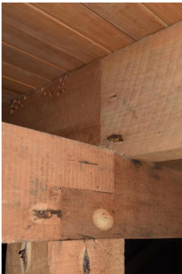
Figures: 6 & 7- Untreated tōtara subfloor framing of houses built in 1953 & 1962. No evidence of borer was observed. N.B. – the distinct colour variation on the same piece of timber (– notably the angled brace in the right-hand image) presumably indicates a transition zone from heartwood to sapwood timber.
