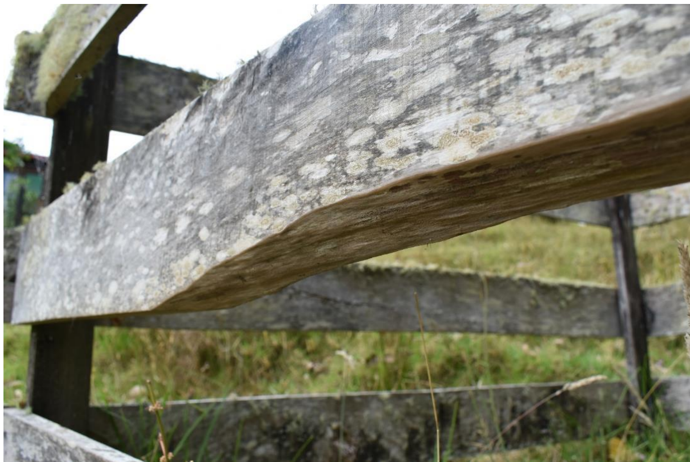
Figure: 18 – Untreated tōtara timber rails milled in 2008 and used in service outside since 2009 (i.e. 7 years so far). N.B. - many boards have wane and will therefore include a portion of sapwood. Although not expected to be durable in this exposed exterior application, no evidence of borer or rot/deterioration is yet evident.
