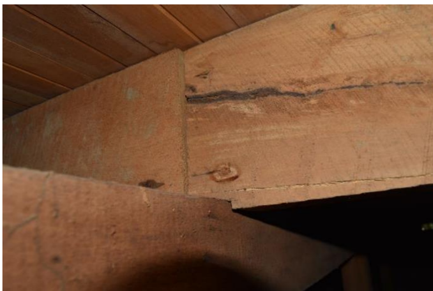
Figure: 8 – Bark encasement on one of the timber joists is presumably associated with a portion of sapwood content on this piece of timber. No evidence of borer was observed.
