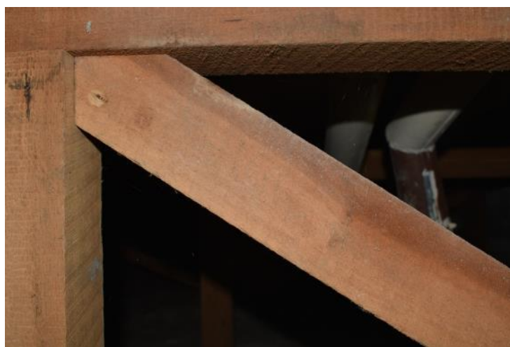
Figures: 6 & 7- Untreated tōtara subfloor framing of houses built in 1953 & 1962. No evidence of borer was observed. N.B. – the distinct colour variation on the same piece of timber (– notably the angled brace in the right-hand image) presumably indicates a transition zone from heartwood to sapwood timber.
