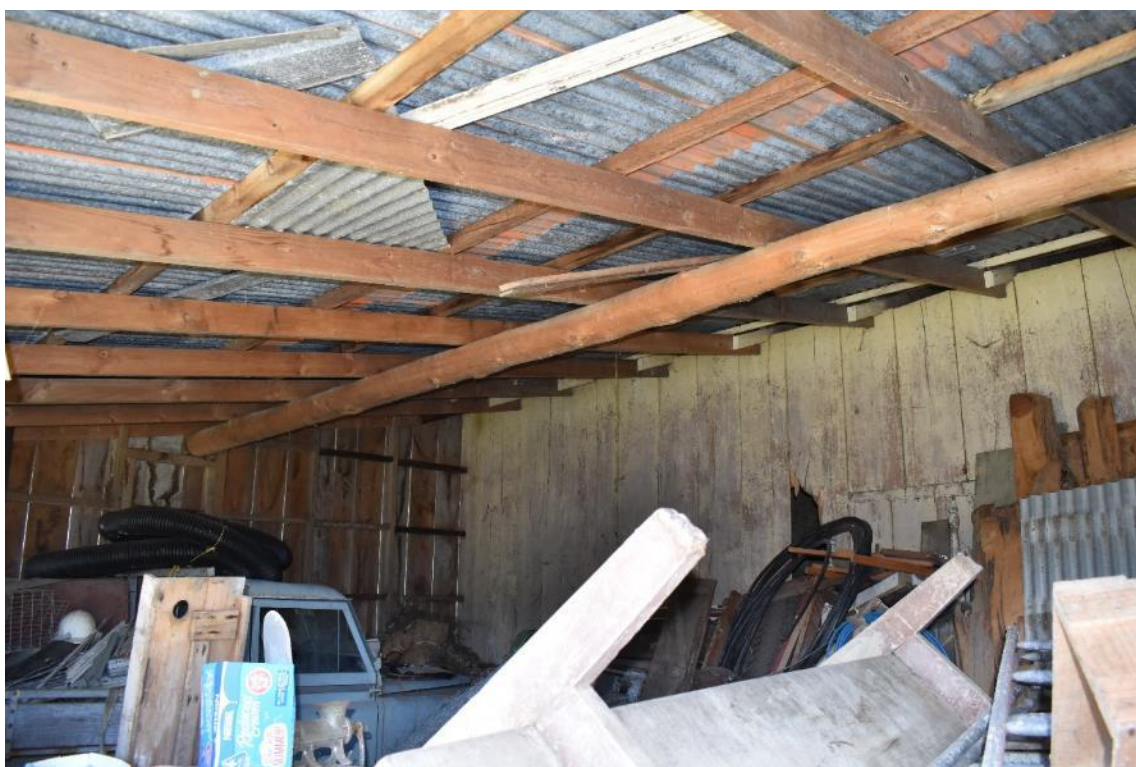
Figure: 21 The 8.57m long beam (under the rafters) has provided the mid-span rafter support since Oct. 1968, is an untreated tōtara pole, mostly still in the round form, but partly flat-sided (by axe) on top and near the butt end. The small end diameter is 160mm and the large end diameter is estimated at <30cm. The beam had the bark removed and was used green. Although borer is present in other timbers in the shed, no borer attack was observed at all in this (or the other) tōtara beam.
