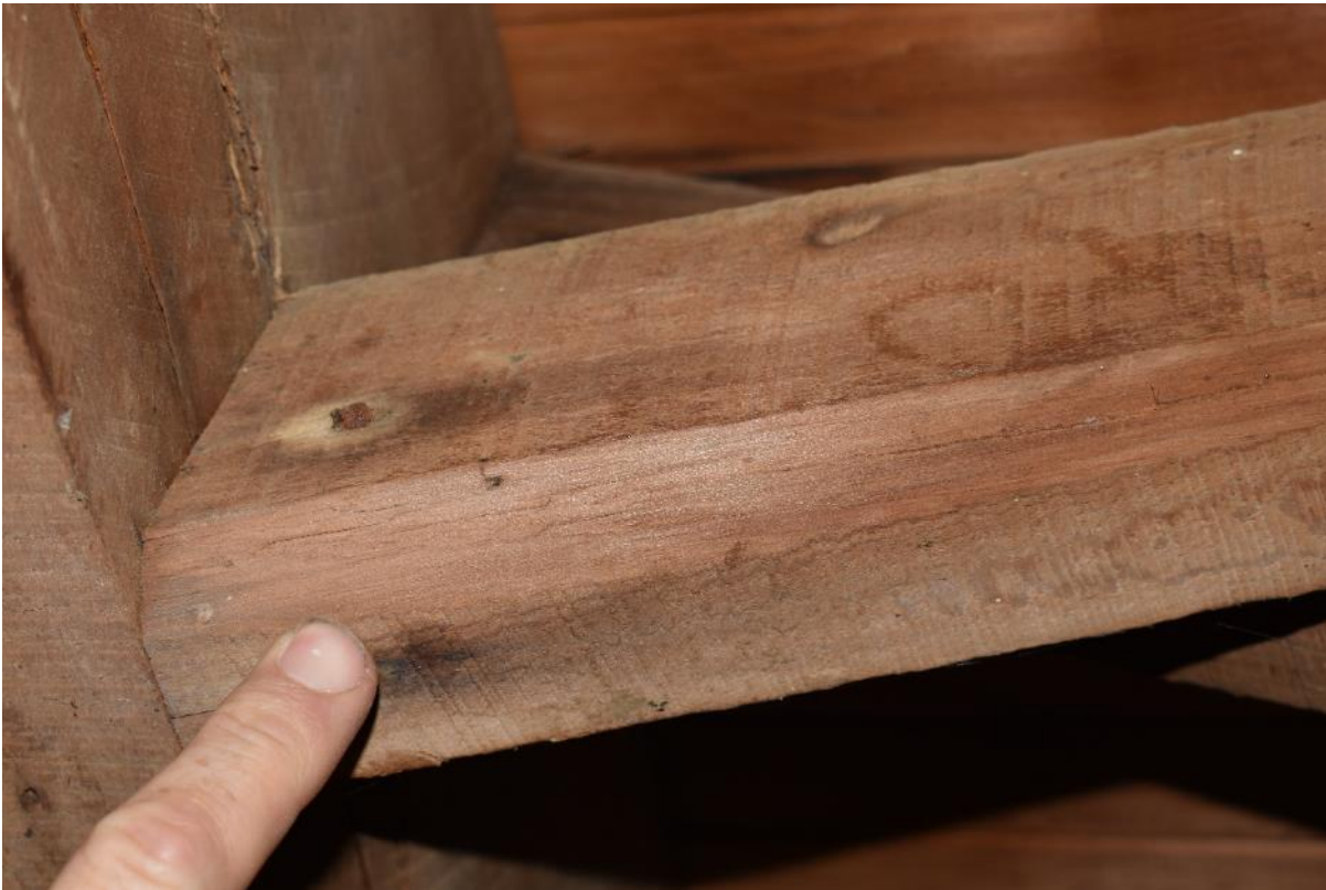
Figure: 9 – Obvious incidence of wane indicates the definite presence of sapwood on this piece of timber (in service since 1953). No evidence of borer was observed.
