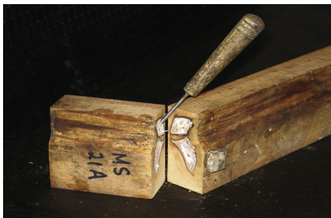
Fig. 7. The joint surfaces in treated macrocarpa where preservative penetration was incomplete, after 18 months exposure in an enclosed tank. There was no decay on the outside of this sample but there was severe internal decay in the sapwood.
