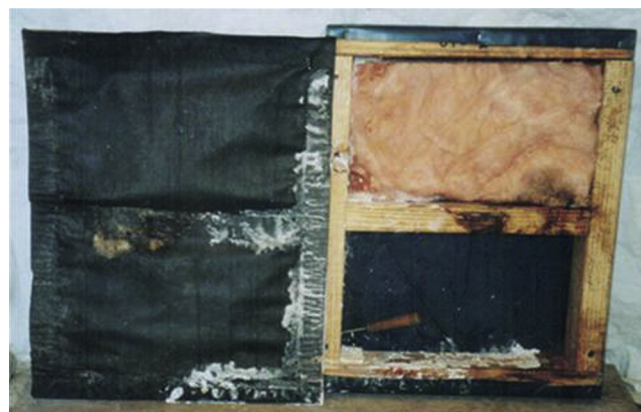
Fig. 3. An untreated wall unit after twelve weeks exposure. The fibreglass insulation has been removed from the lower half to allow assessment of decay. Mycelium from the O. placenta feeder blocks (on the left) was spreading through the fibreglass insulation and on the surfaces of the framing. C. puteana mycelium (on the right) had spread up the right stud across the dwang into the fibreglass and across the building paper.
