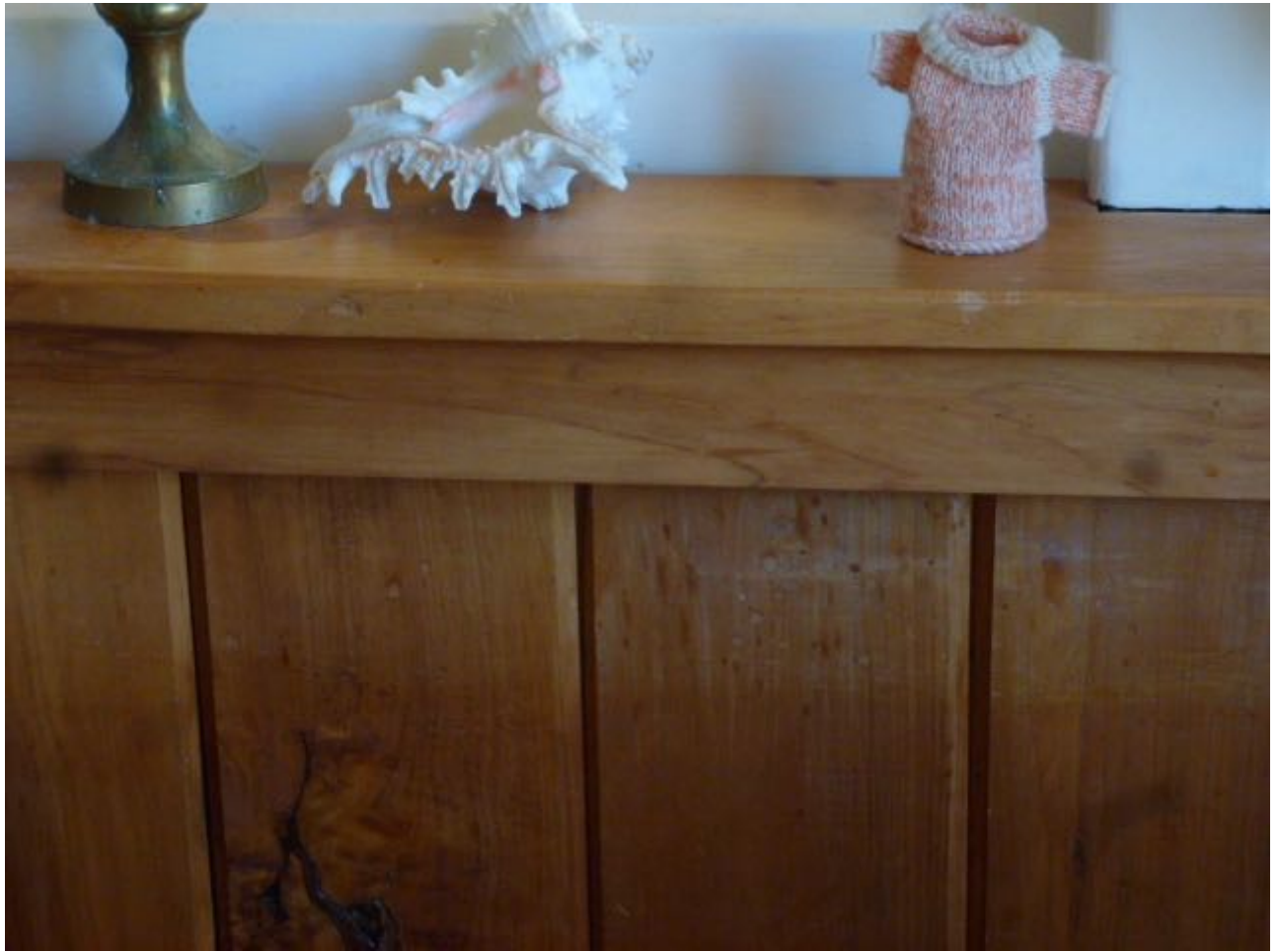
Interior shelving above sarking (with evidence of household activity but no borer)
