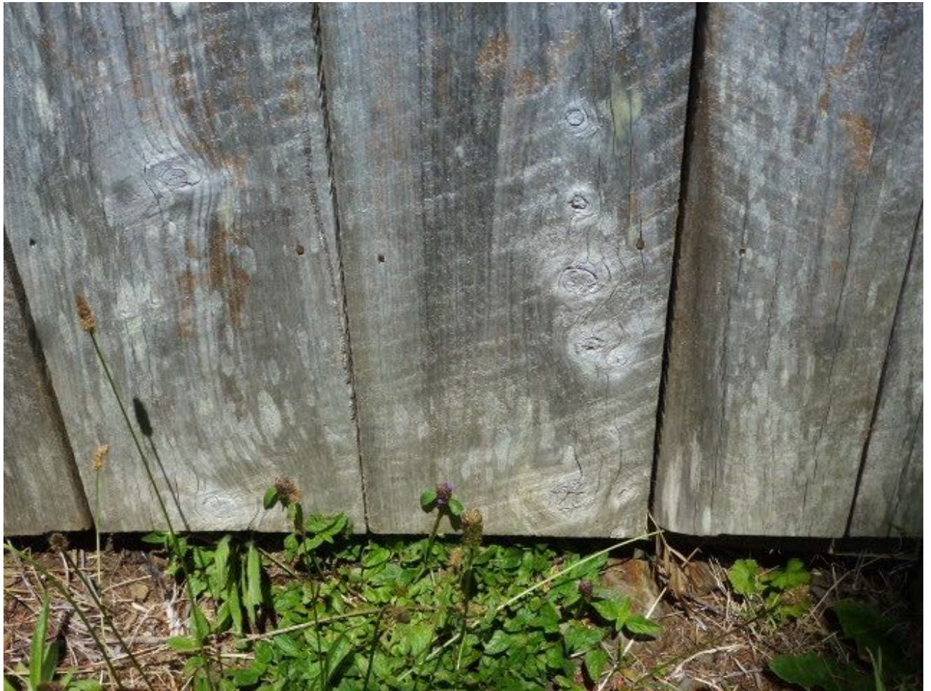
Detail of footing showing no rot.
