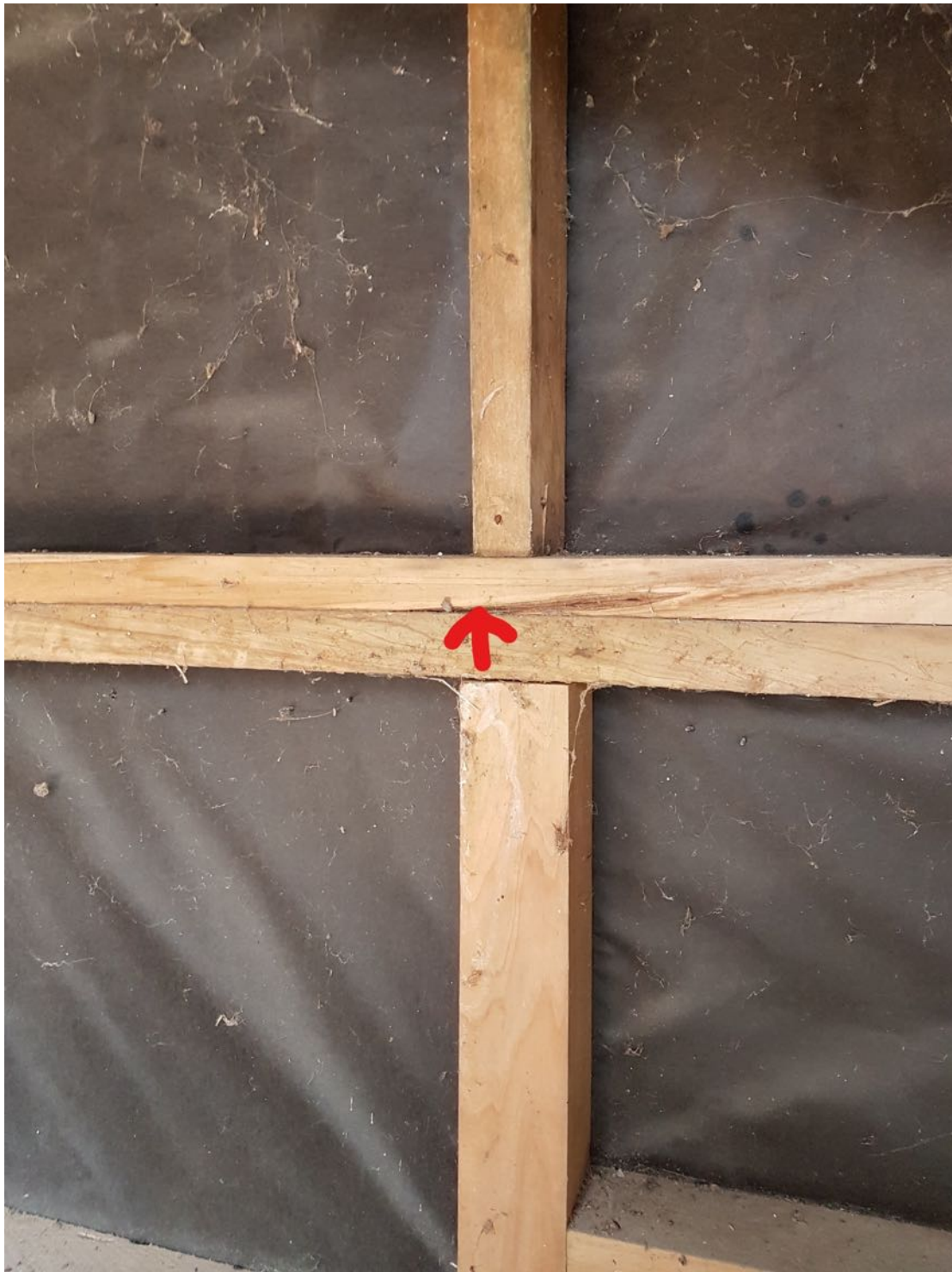
Cypress framing showing sapwood with bark encasement. No borer present.
