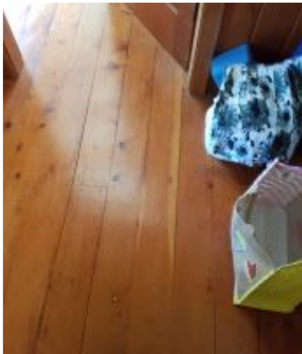
Macrocarpa floor over joists showing sapwood
