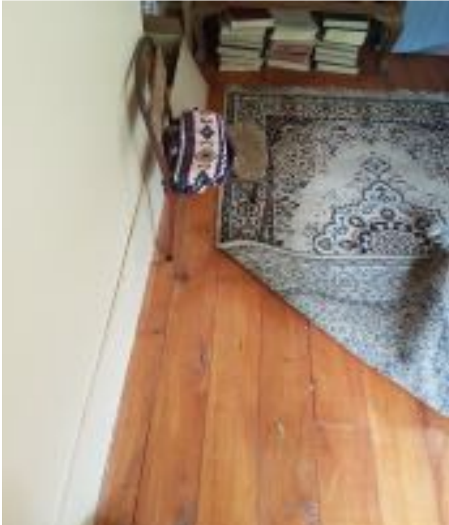
Macrocarpa floor over joists showing sapwood
