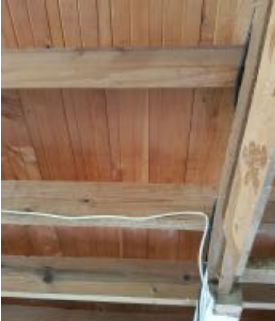
Macrocarpa upstairs floor from below showing sapwood
