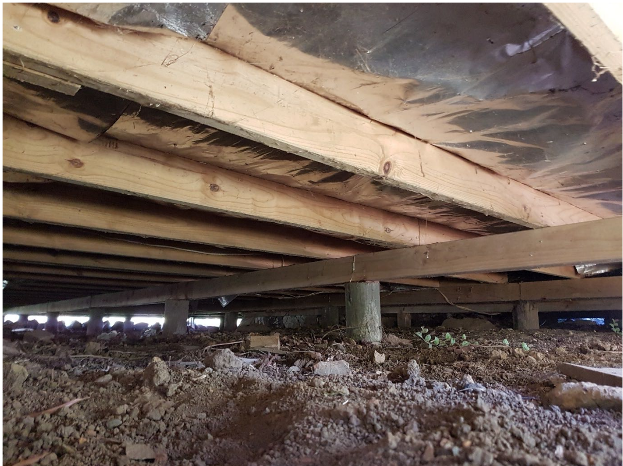
Macrocarpa floor over joists. Piles under floor range from less than 300ml to 600ml above ground
