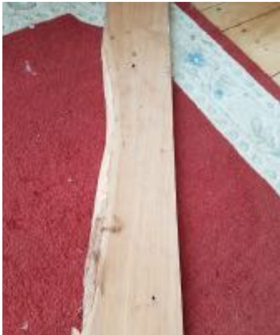
Macrocarpa sapwood removed from building for inspection. No borer present, just nail holes.
