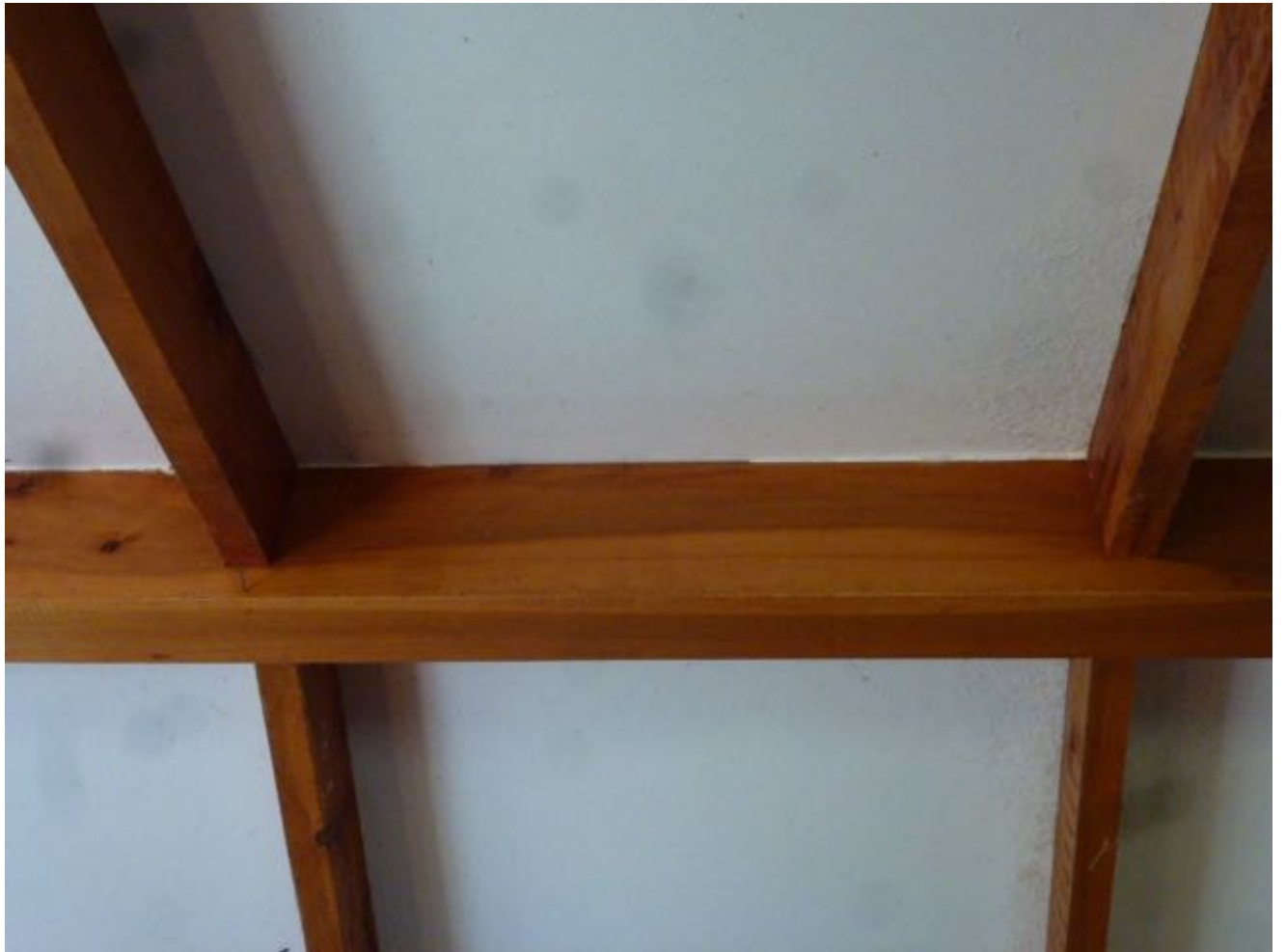
8" x 4" beam with rafters showing sapwood
