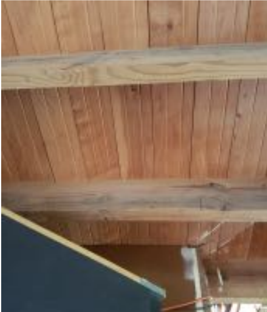
Macrocarpa upstairs floor from below showing sapwood
