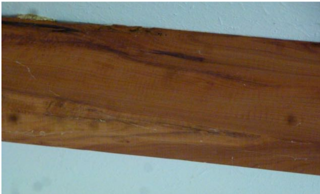
6" x 2" macrocarpa rafter showing sapwood
