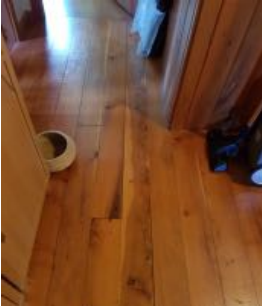
Macrocarpa floor over joists showing sapwood
